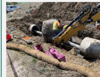
Camp Stoneman Interceptor Repair
