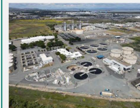
District's Wastewater Treatment Plant
