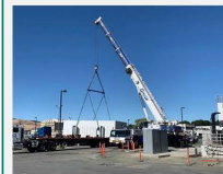
Delivery of New Electrical Switchgear
