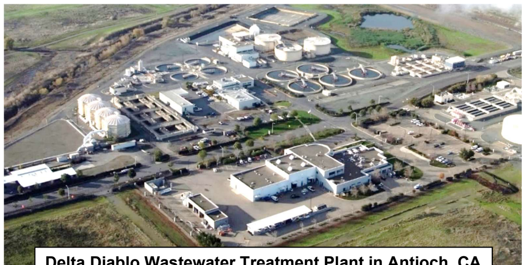
Delta Diablo Wastewater Treatment Plant in Antioch, CA
