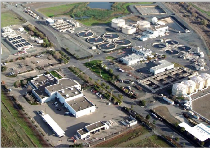
TREATMENT PLANT AND DISTRICT OFFICES
