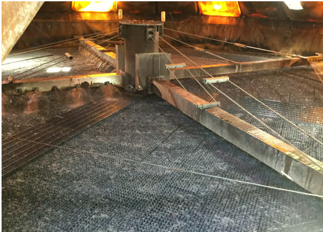
Figure 2-1 Delta Diablo Tower Trickling Filter Media
