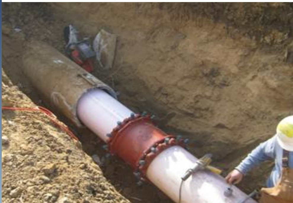
Pittsburg Pipeline Rehabilitation
