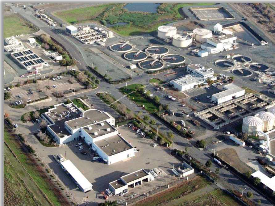
Treatment Plant and District Offices
