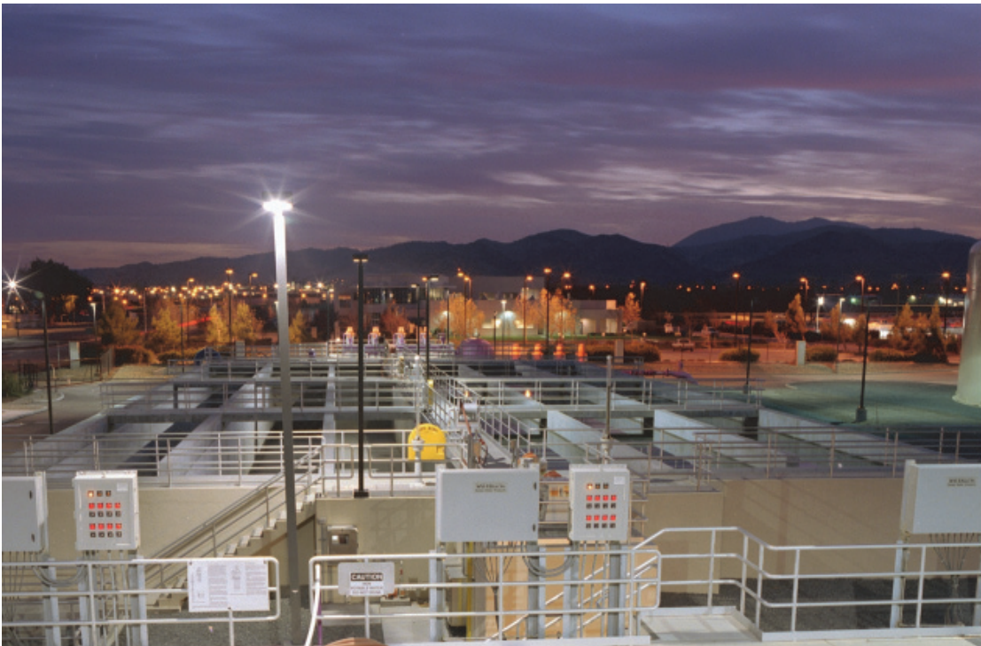
Recycled Water Facility – Chlorine Contact Tanks
